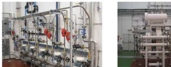
Electrolyzer (1600mm) in FHA facilities
