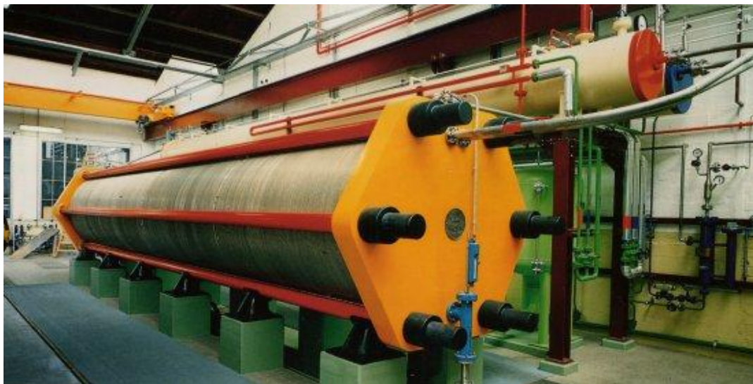
Figure: Picture of the Type S-556 electrolyser of IHT
